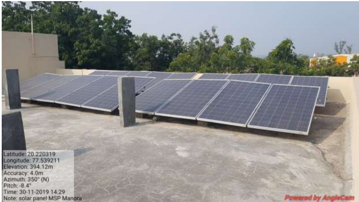
5.5 kW Solar Panel on hostel Roof of college
