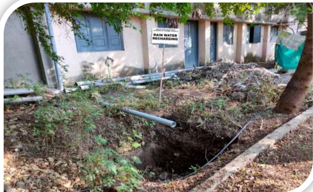
Rain Water Recharging pit
